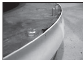
Planetary seal - closeup
